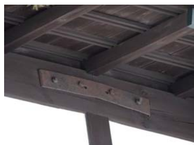
桁継手の帯金物補強
